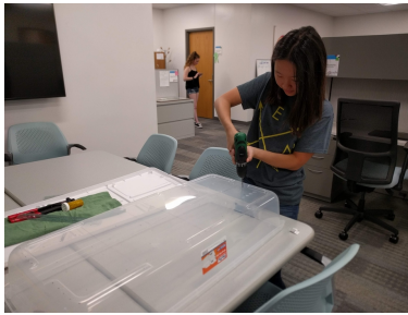
Figure 1: Drilling holes into the bin will allow water to drain out of the apparatus
